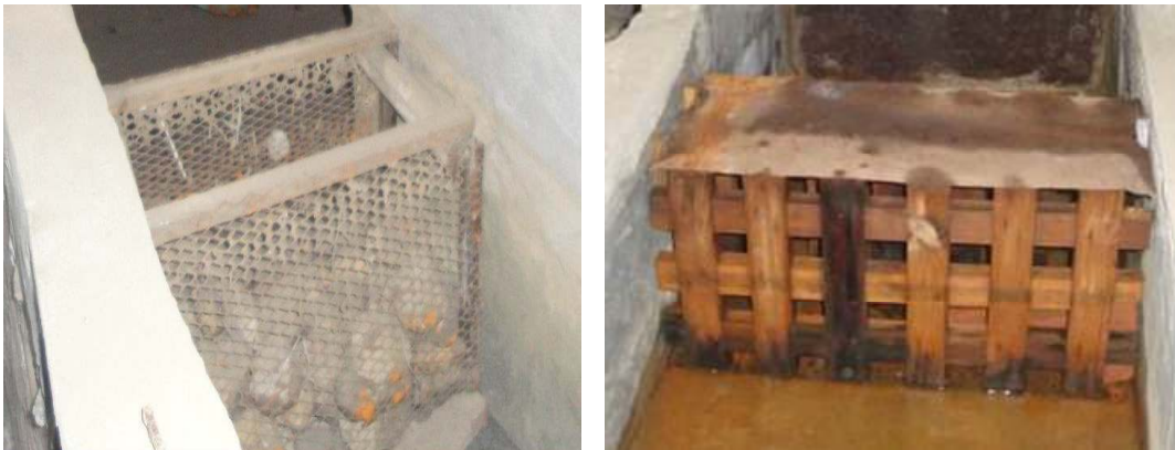
Fig. 4. Screen stone and wooden boxes
