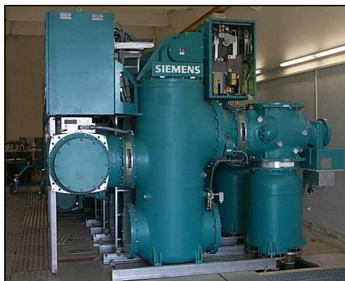
Figure 1: Compact design of 145 kV GIS
